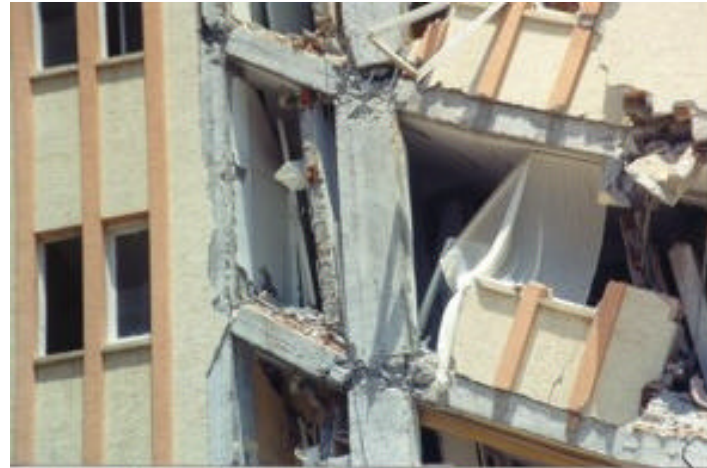
Beam-column failure
